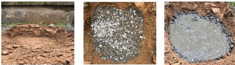
Fig. 5 Base Preparation for Casting Area
